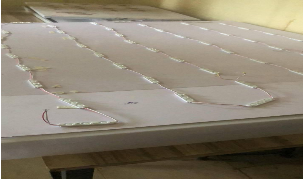
Fig: 8 Installation Of LED Lights
