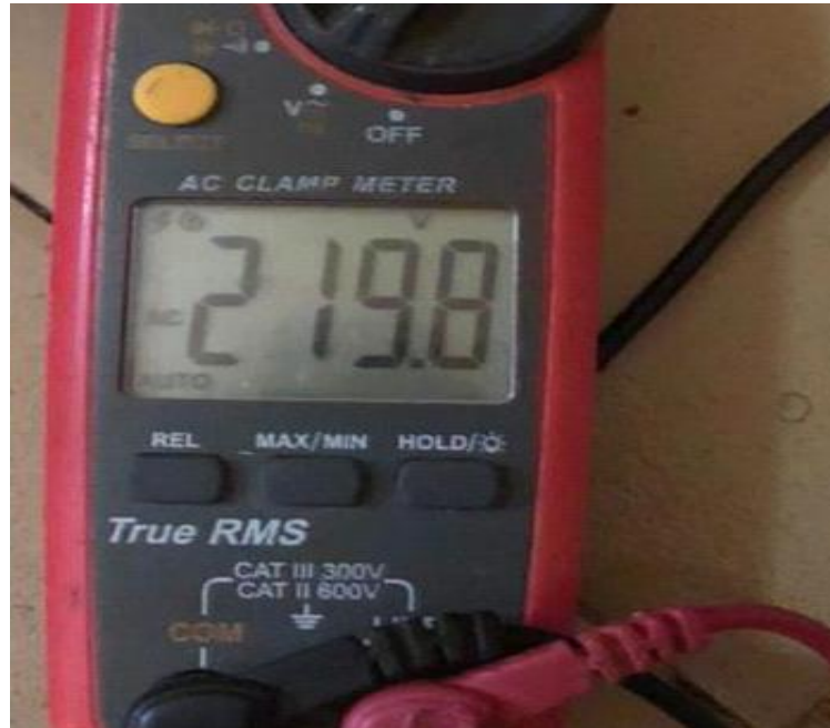
Figure 4.13: OUTPUT VOLTAGE TEST FOR LOCAL INVERTER
