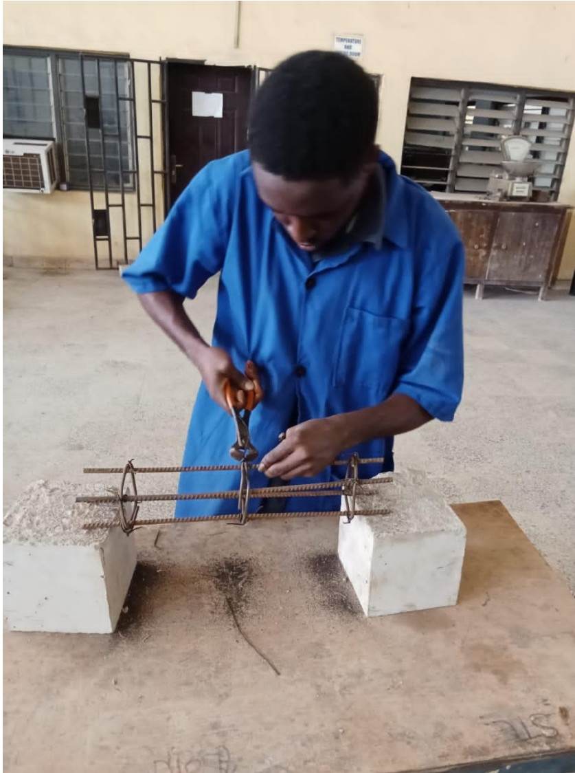
Binding of steel rods
