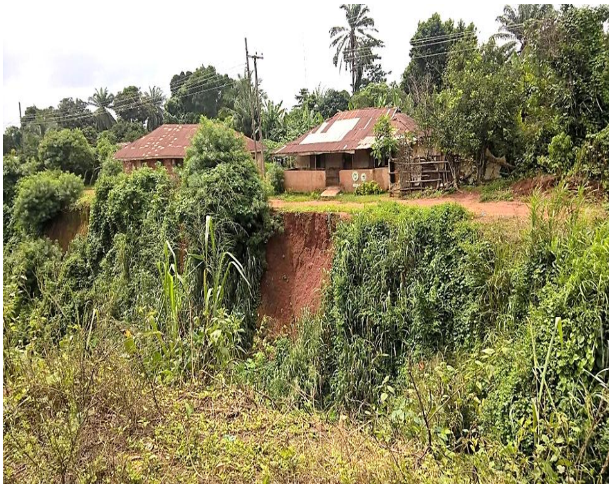
Plate 3.2: The back view of the gully erosion site in Evbhomore community in Ovia North East Local Government Area of Edo State
