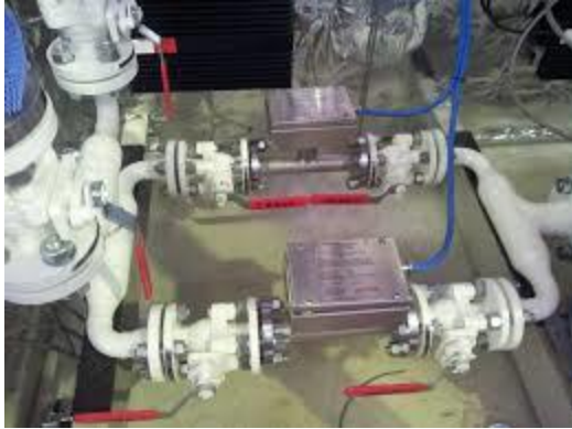
Figure 1.2: BS&W Probes for LACT Units (Eesiflo Technologies)
