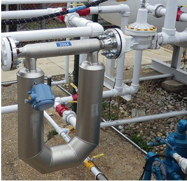
Figure 1.1.3: Coriolis mass flow meter (Modern Pumping Today)
