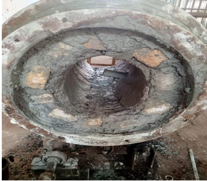
Figure 3.6: Ongoing Casting of the Rotary Furnace
