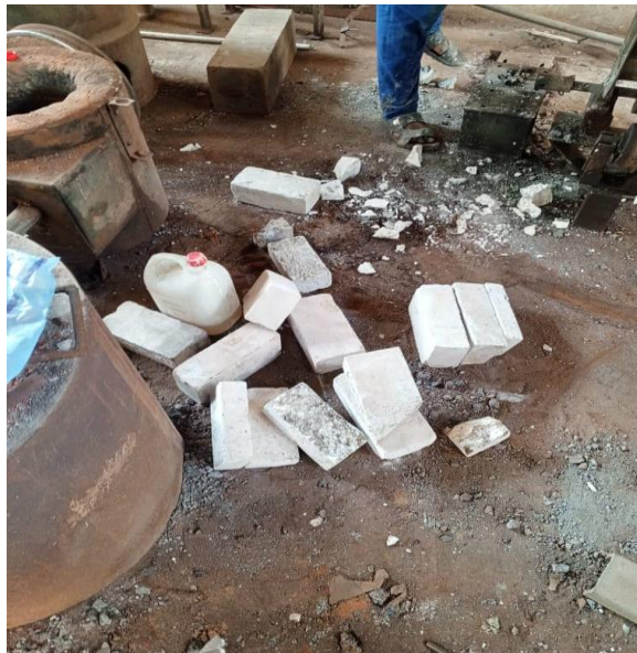
Figure 3.1: Preparation of Materials for the Casting of the Furnace
