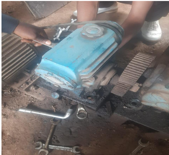
Figure 3.3: Uninstallation of the Electric Motors for Offsite Repairs
