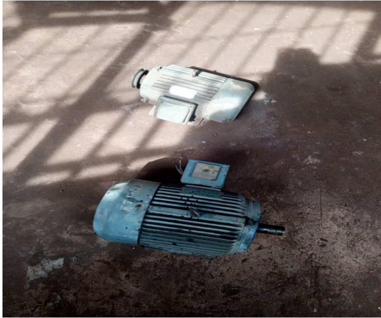
Figure 3.4: The Electric Motors on the Ground after Removal from the Base
