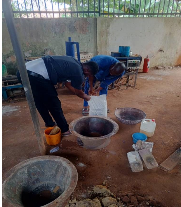
Figure 3.2: Continued Preparation of Materials for the Casting of the Furnace
