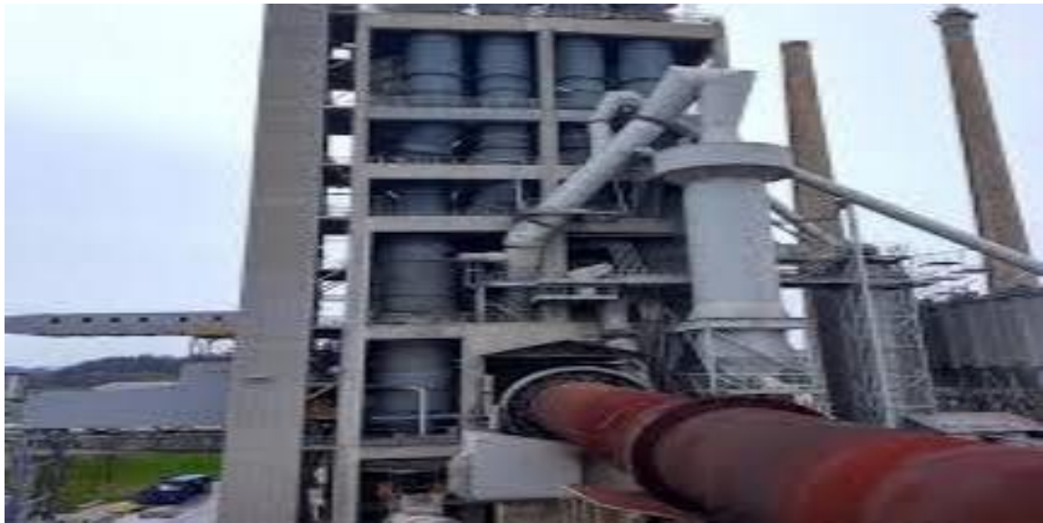
Figure 2.3 Pyro Process of the cement ;( Bua cement plant. 2025)
