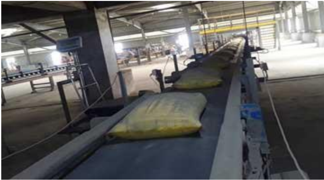
Figure 2.9 Packaging section (Bua Cement, 2025)
