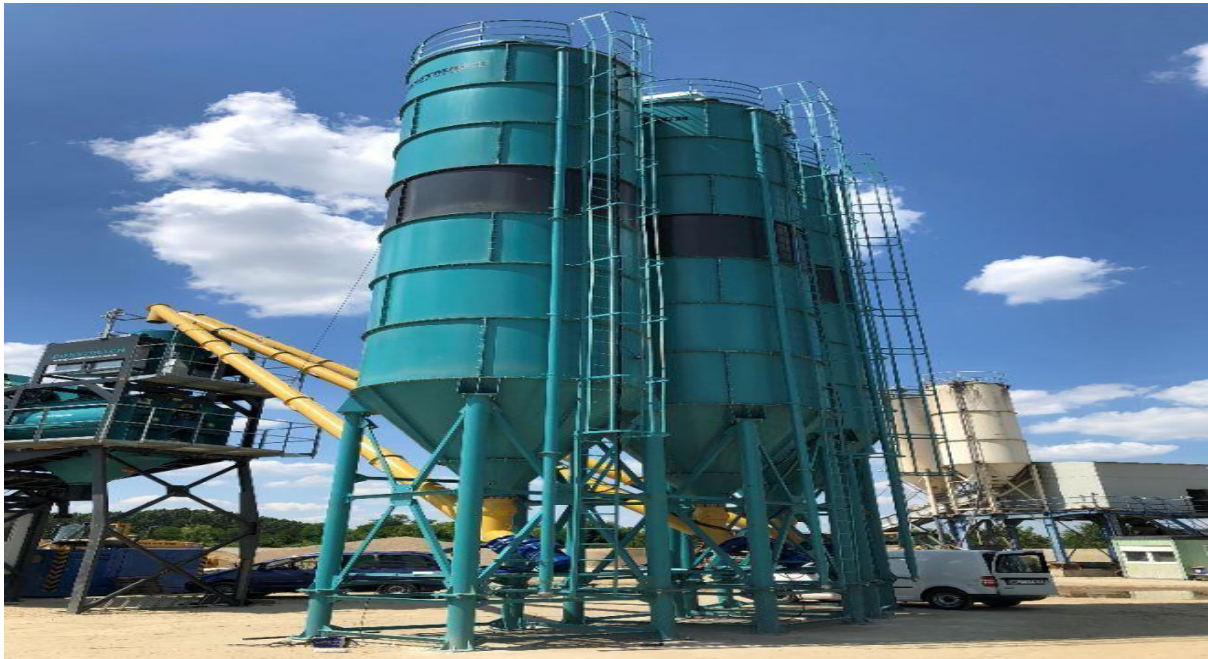
Figure 2.8: Cement Silos ;( CMQ Engineering)
