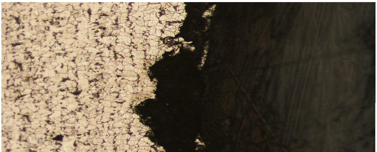
Figure 4.9: Pitting corrosion on the OD of the affected area.
