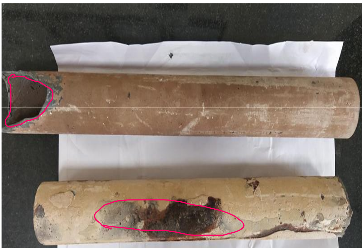
Figure 4.6: Fractured Sample collected for further analysis
