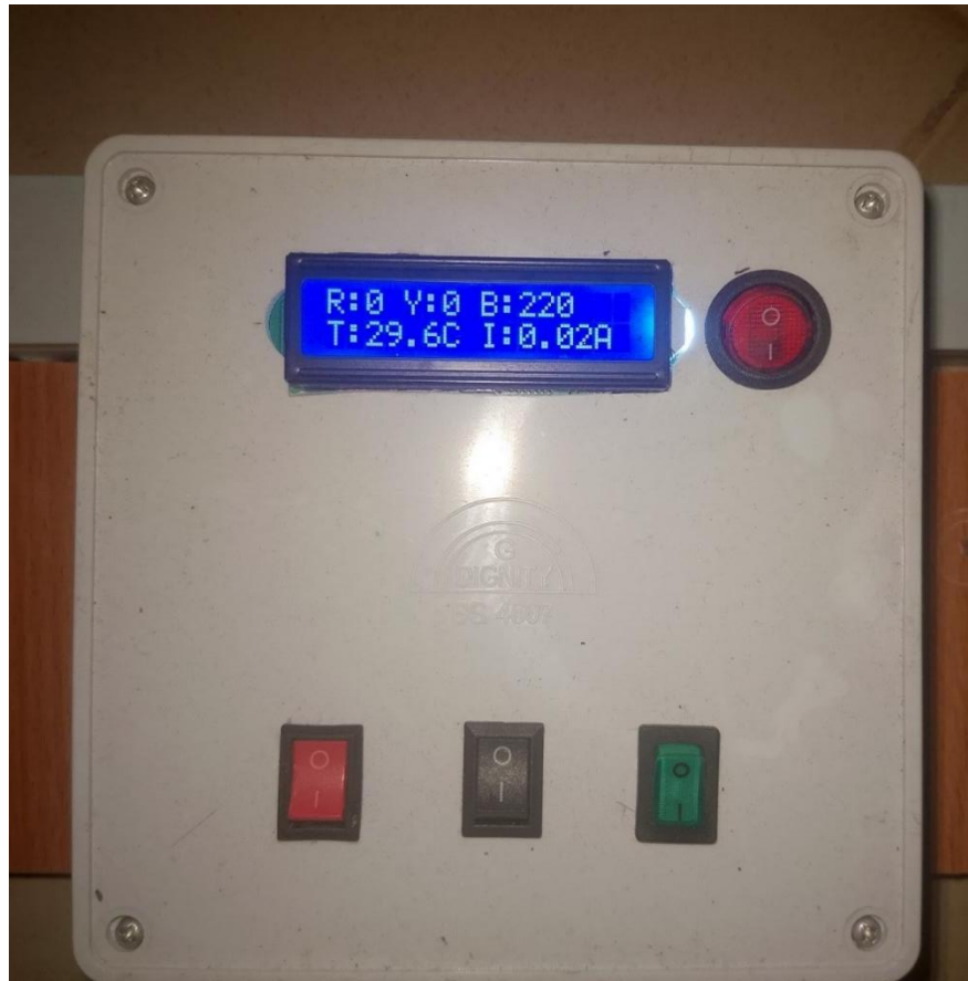
Figure 4.6 Voltages Applied To Each Phase Being Read
