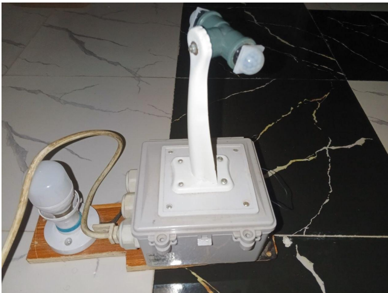
Figure 4.3: Complete PIR Sensor Setup
