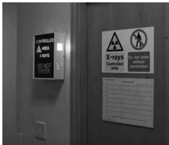
Figure 2.5: Entrance to a controlled area showing warning signs and lights.
