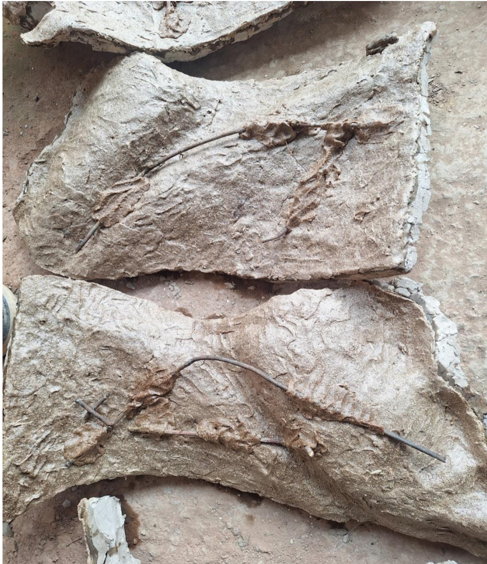
Iron rod reinforcement Photographed by John Anabui Year: 2025
