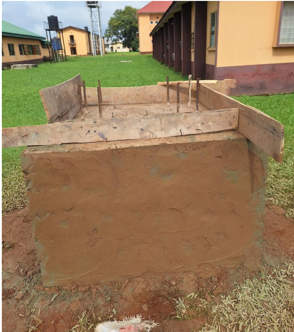
Step Casting Photographed by John Anabui Year: 2025
