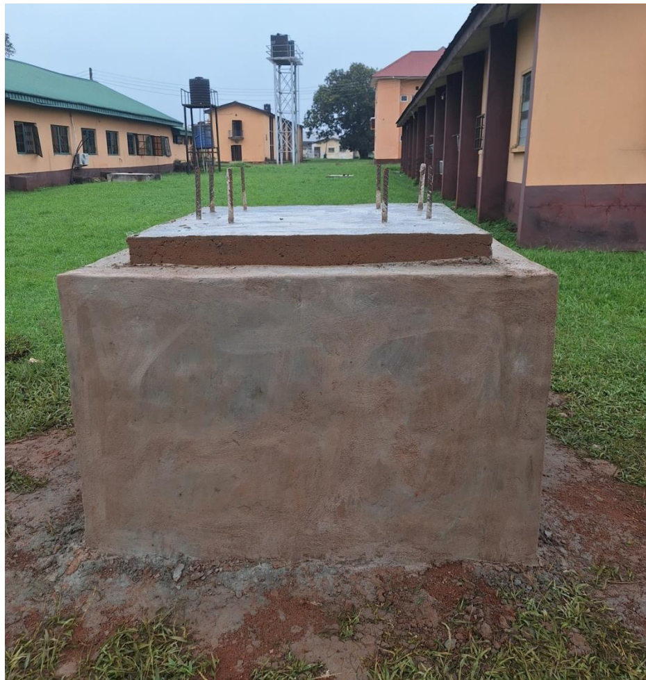
Completion of the plinth Photographed by John Anabui Year: 2025
