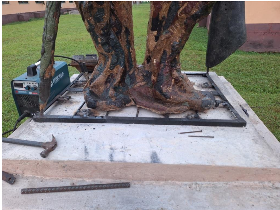
Welding of the Sculpture's base to the top of the plinth Photographed by John Anabui Year: 2025
