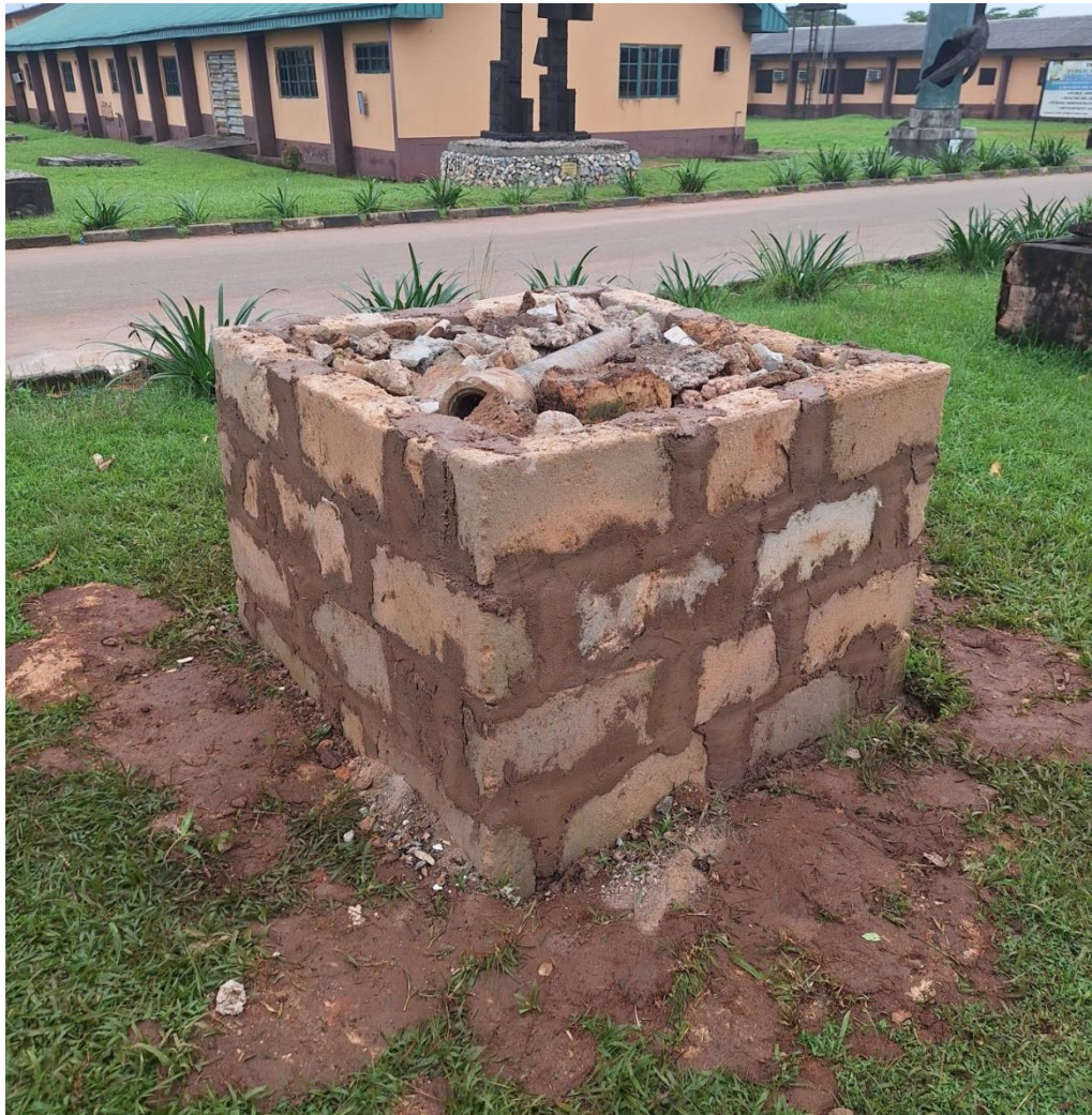
Construction of the Plinth Photographed by John Anabui Year: 2025
