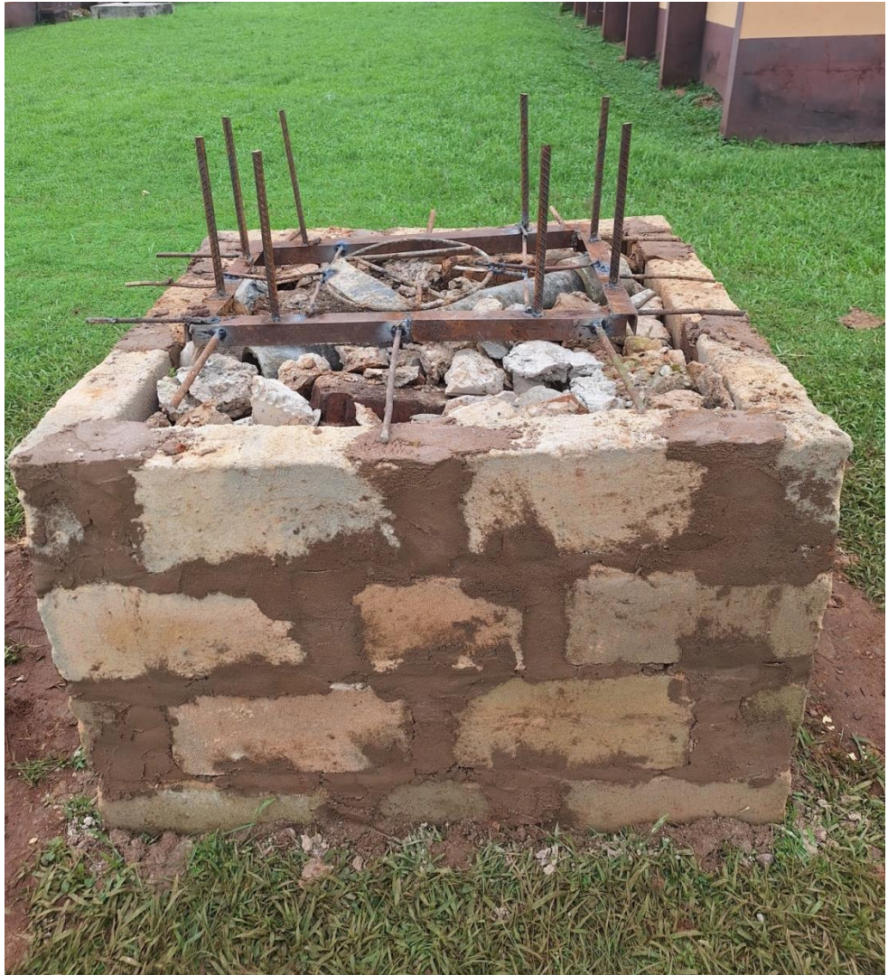
Installation of the iron base Photographed by John Anabui Year: 2025
