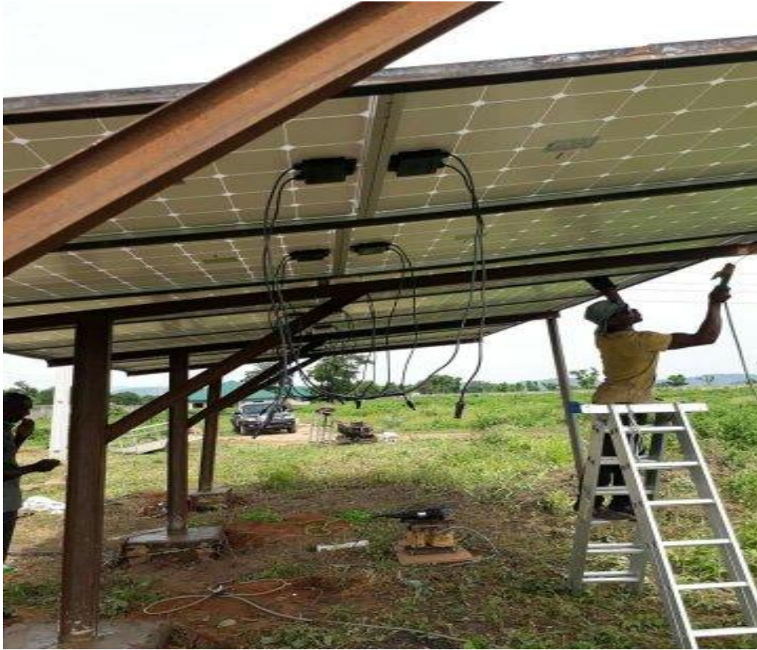
Figure 4. 10: Mounting the Solar Mini Grid
