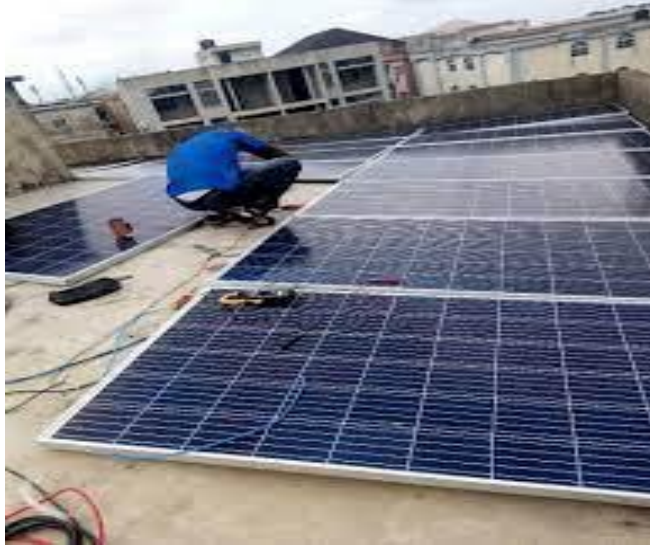
Figure 4. 1: Connecting the Solar Mini Grid
