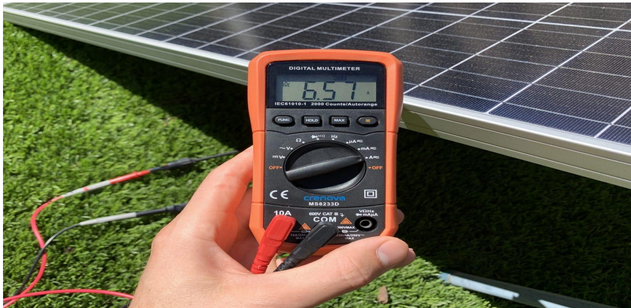
Figure 4. 2: Taking Readings from The Solar Grid
