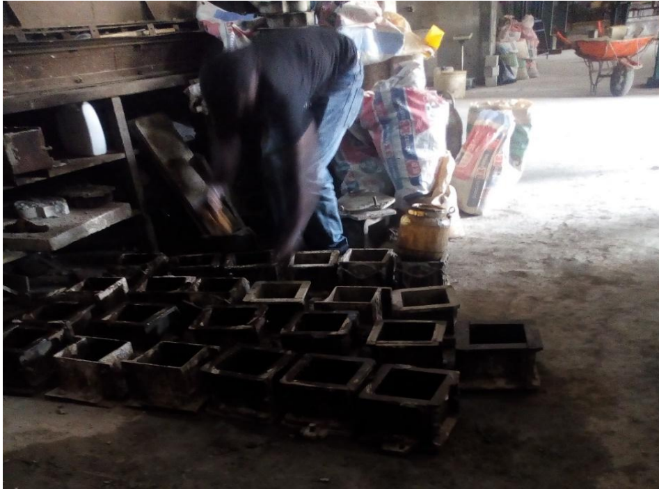
Plate 3: Lubrication of Cube Moulds in preparation for casting
