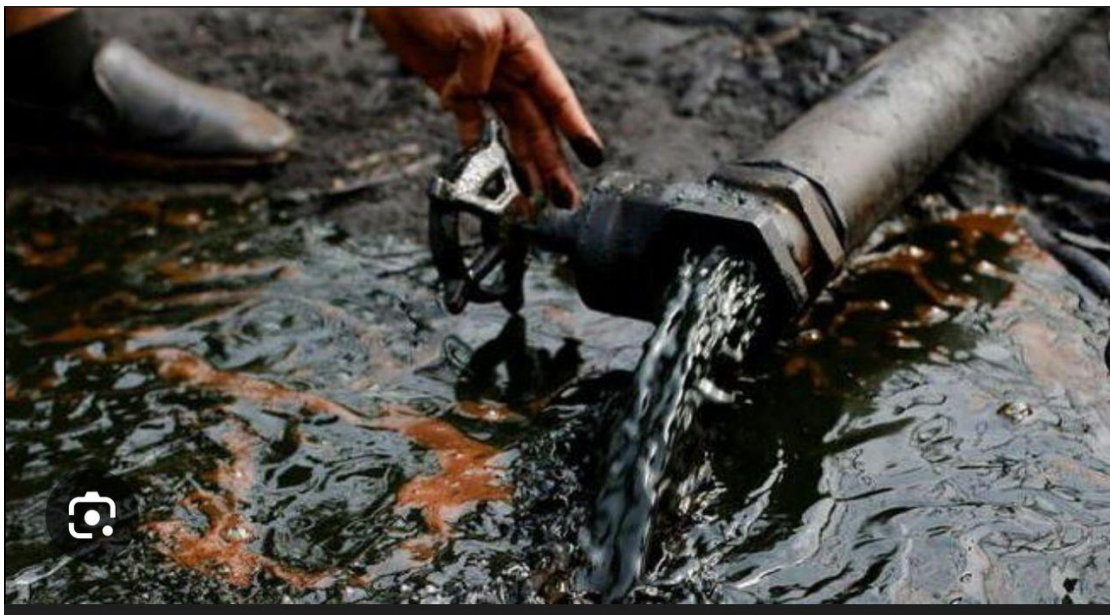
Fig 14: Picture of sabotaged pipeline in the Niger Delta 24
