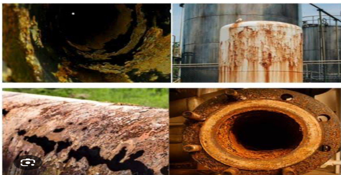
Fig 16: Picture of an Old and Corrosive Pipeline 43
