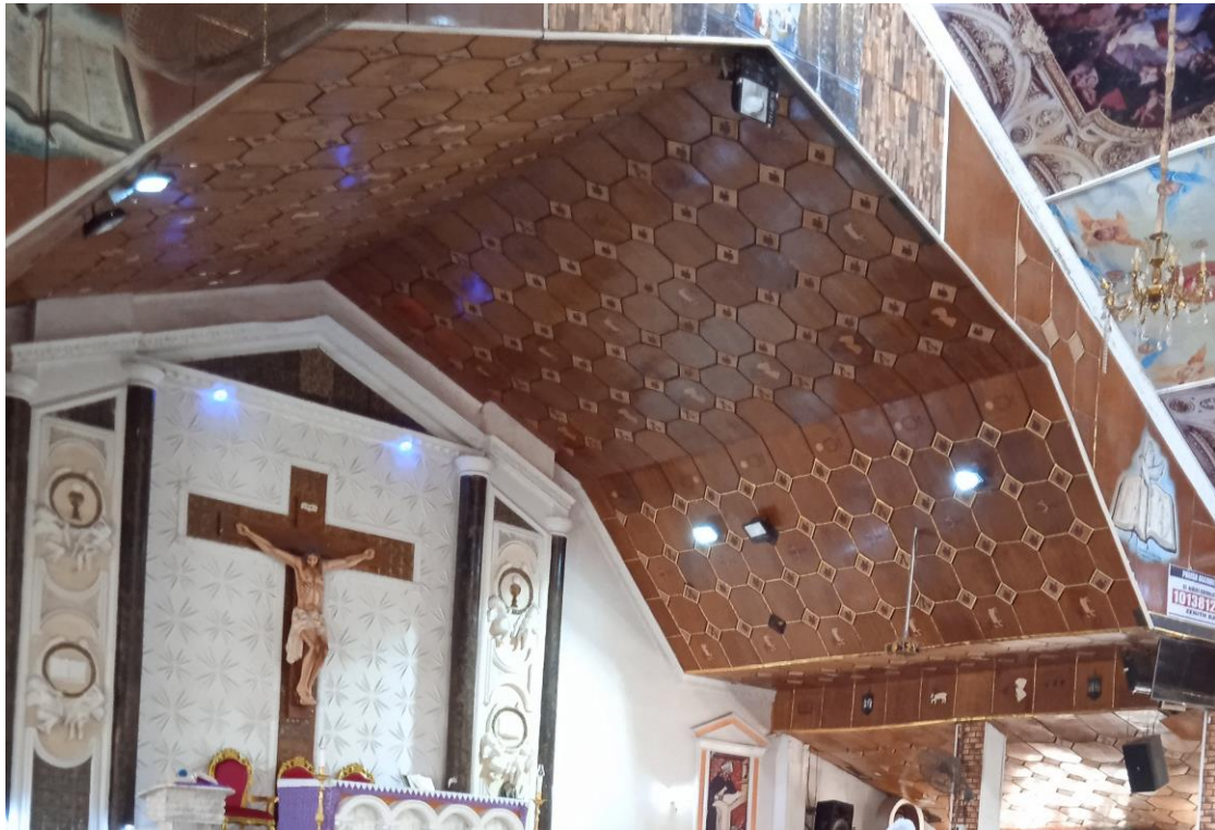
Plate 4: Interior view of the timber ceiling Source: Researcher Field Work (2025).
