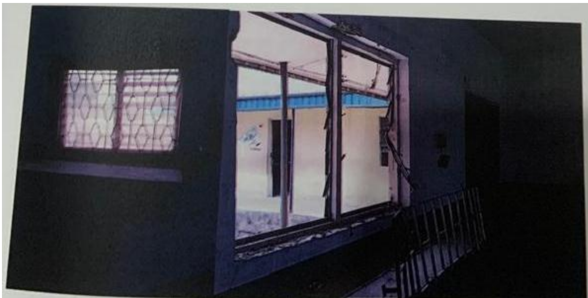
Plate 17. Removal of the old windows
