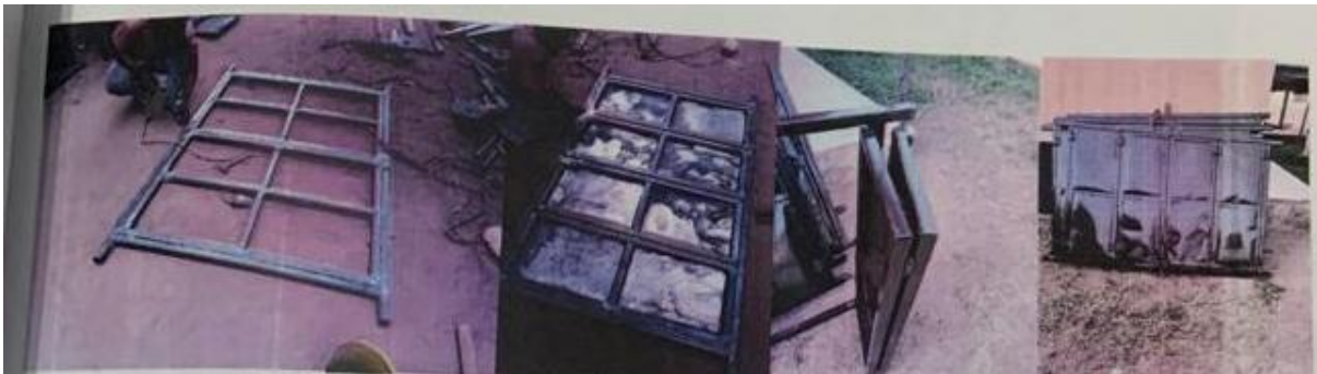
Plate 16. Crafting of the windows at the welders shop
