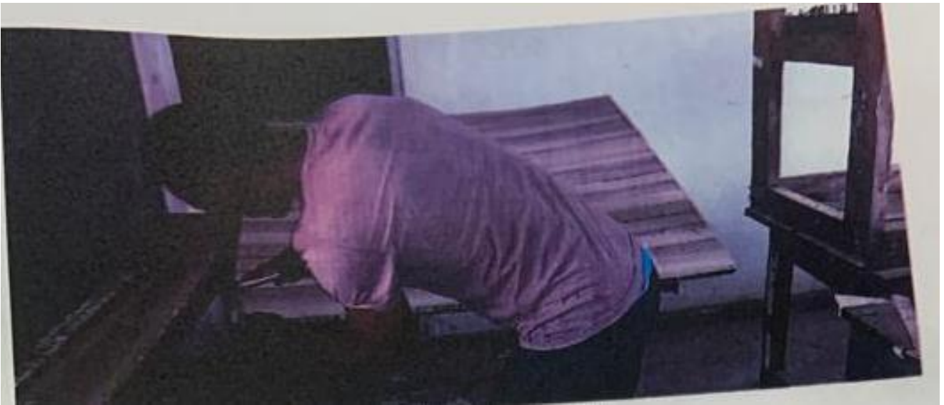
Fixing the boards
