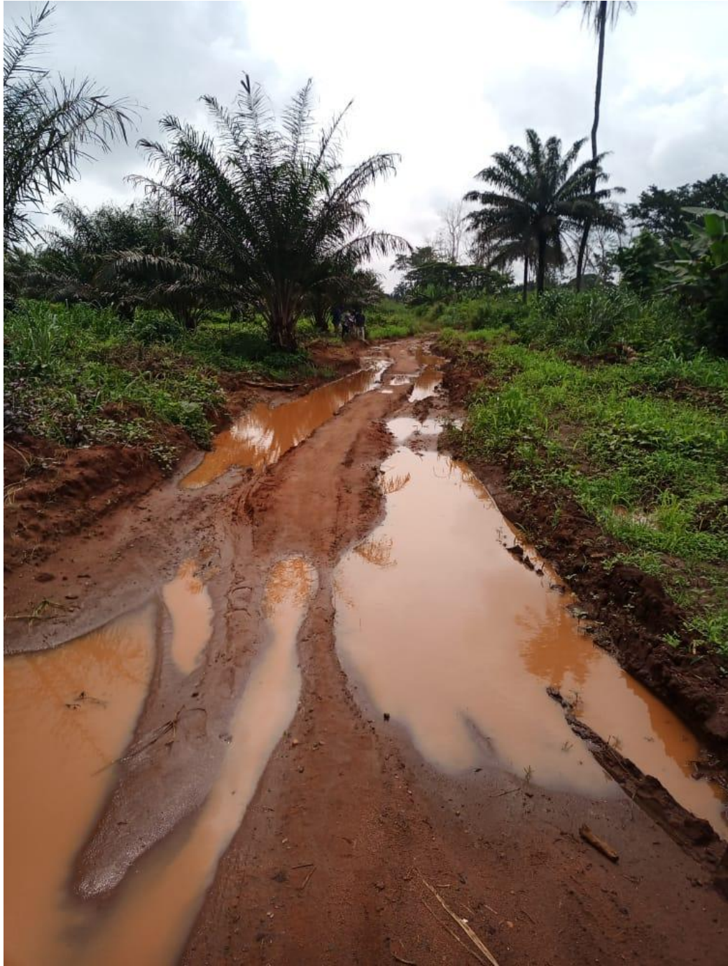
Plate 3.2: Flooded Soil Source: Author's Fieldwork, 2021.
