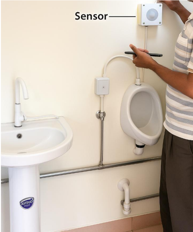
Fig. 3.14: View of Completed Work
