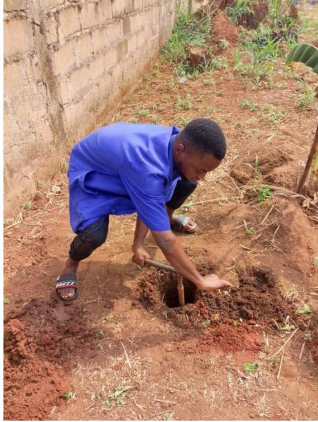
Plate B - 3 Digging a borehole with an auger
