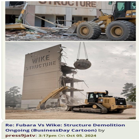
Fig 2 "Structure Demolition ongoing" (BusinessDay, fig.2)
