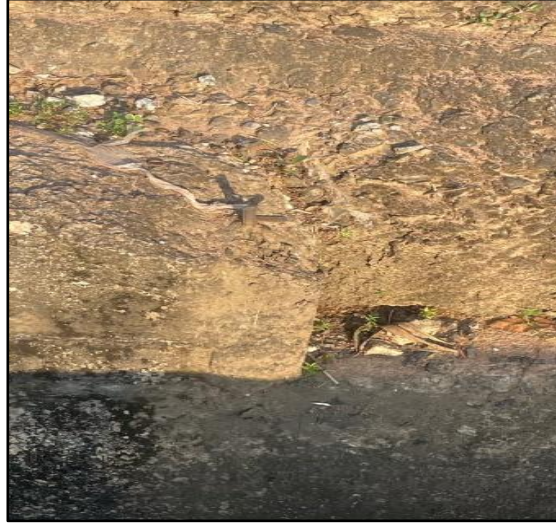
Figure 4.4: Material degradation/ Spalling.
