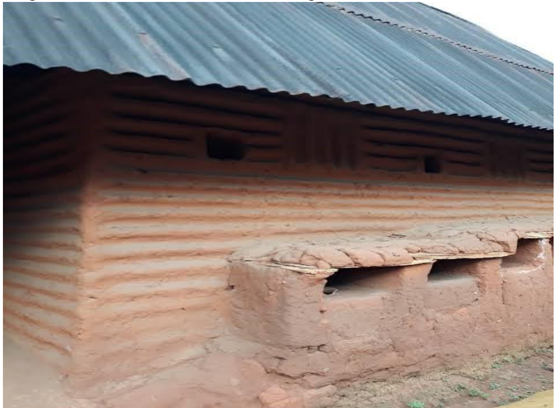
Fig. 18 / Source: Rammed Earth Building Under Construction
