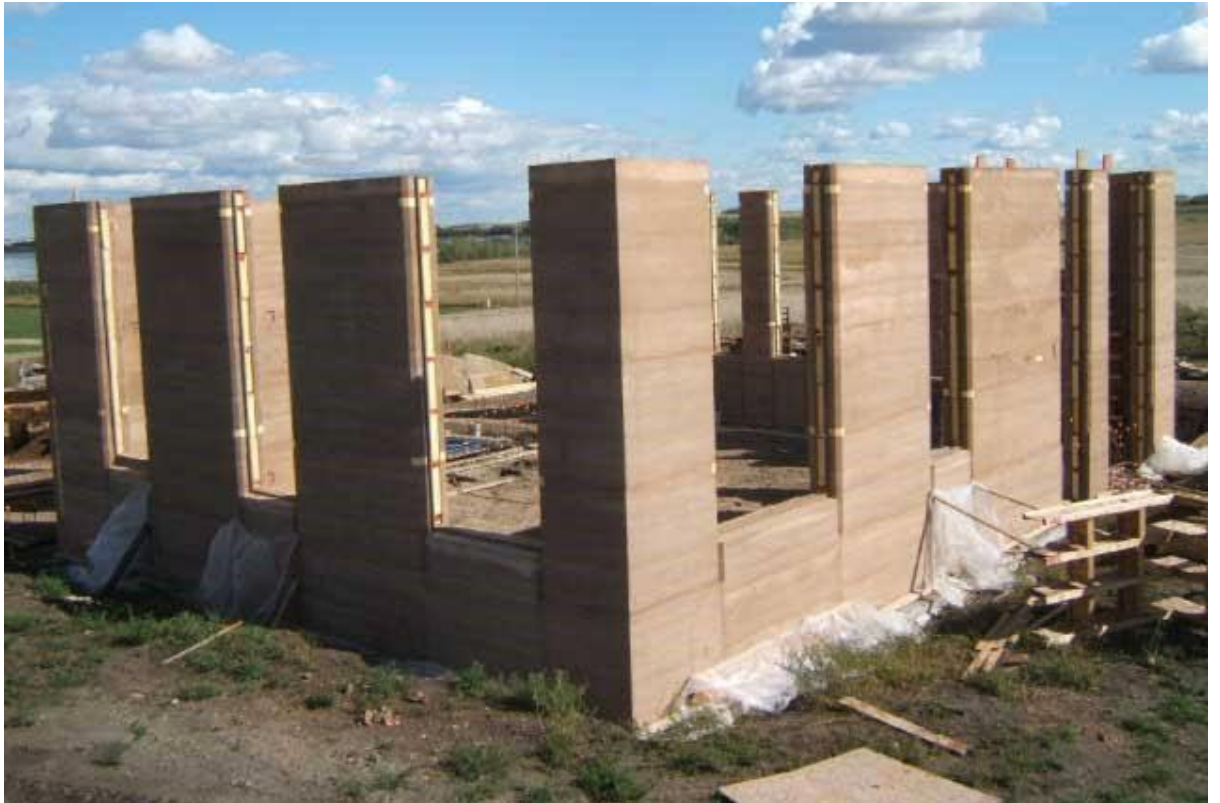
Fig. 17 / Source: Rammed Earth Building Under Construction
