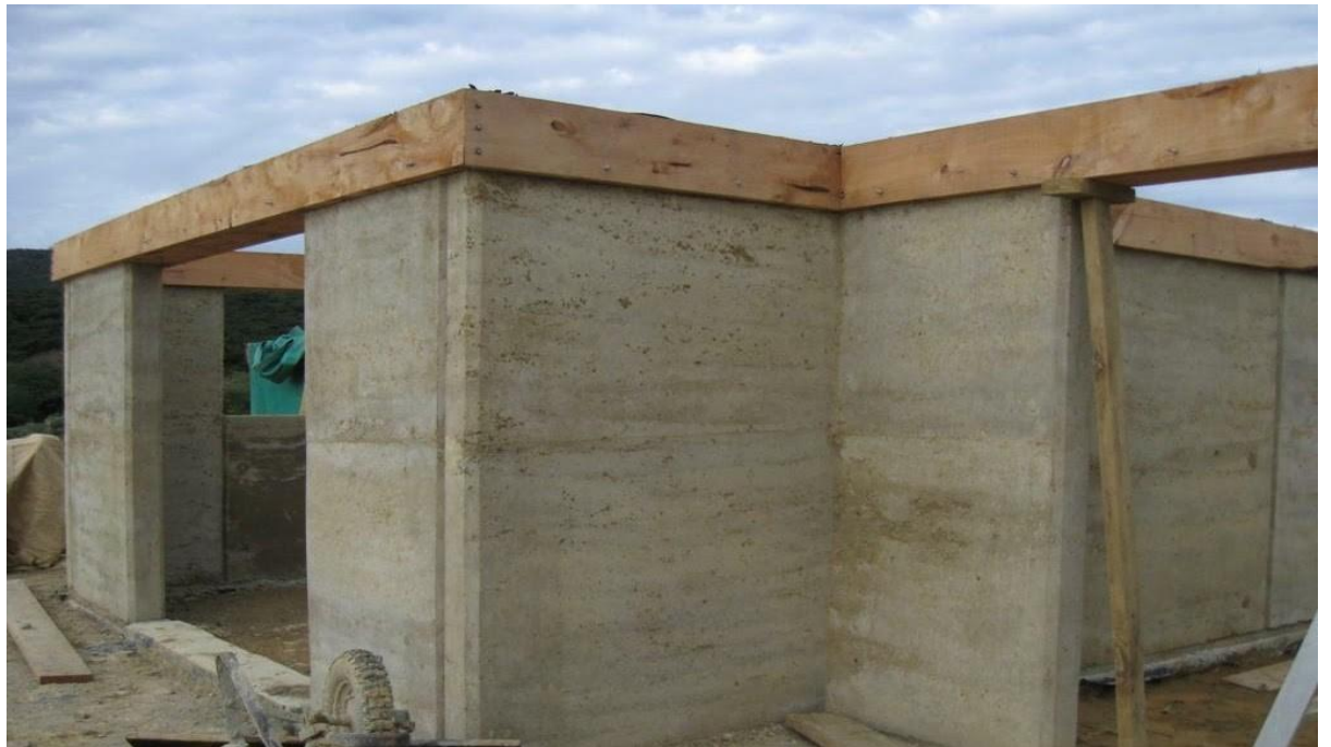
Fig. 16 / Source: Compaction process of Rammed Earth
