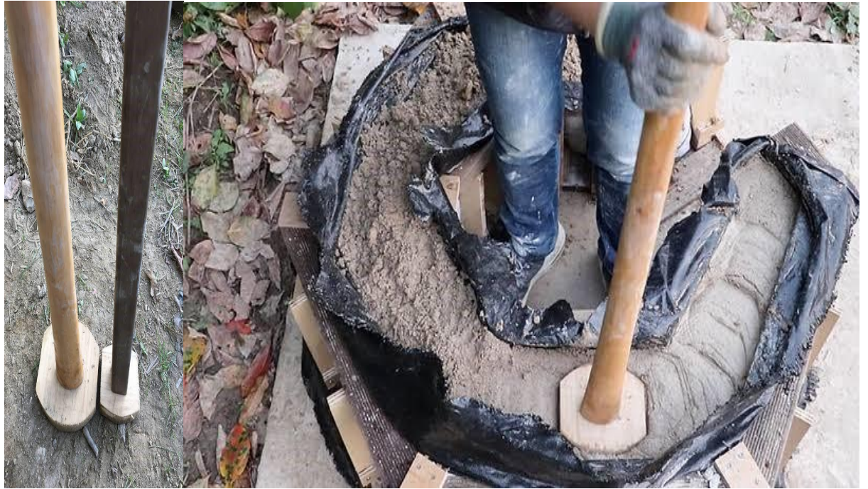
Fig. 16 / Source: Compaction process of Rammed Earth
