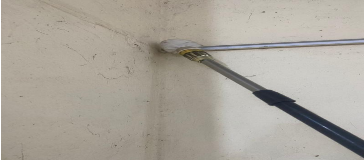
Figure 4.4: Image after cobweb has been removed from painted wall
