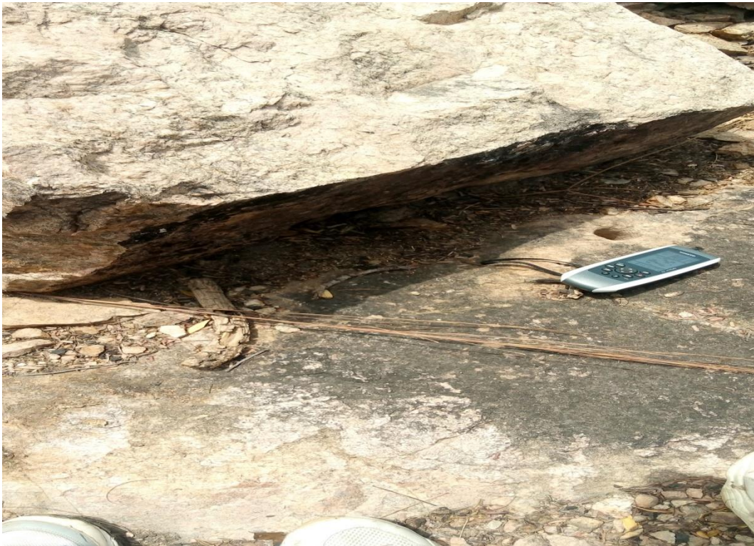
Plate 6: Charged Holes for Blasting
