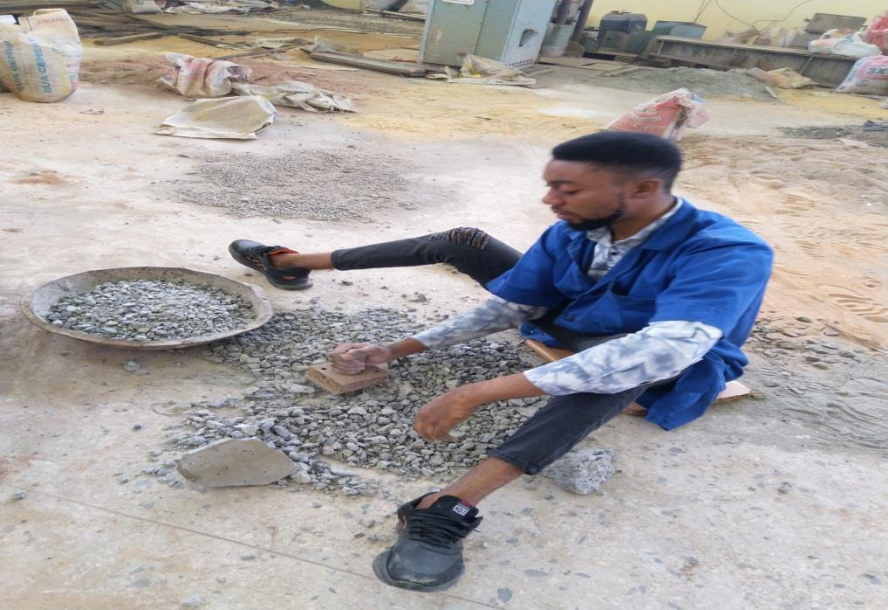
Crushing old concrete
