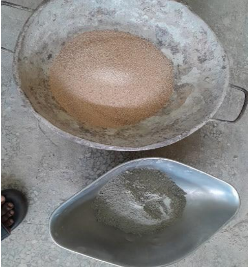
Fig 3.2 graded fine aggregates and weighed cement ready to be mixed
