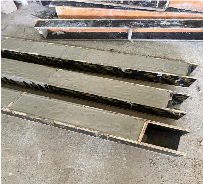
Plate A-5 casting of beams in form works
