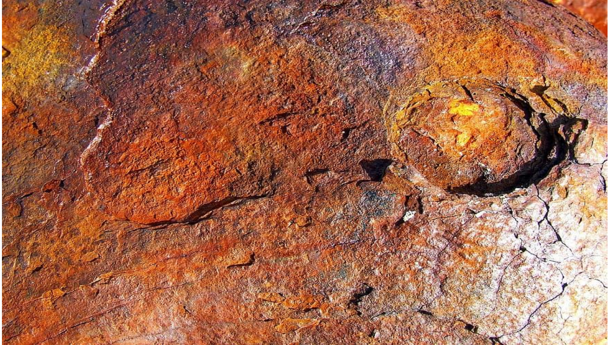
Figure 2.5 The Schematic of General Corrosion of Carbon Steel in Aqueous Environment (pratask, 2009).
