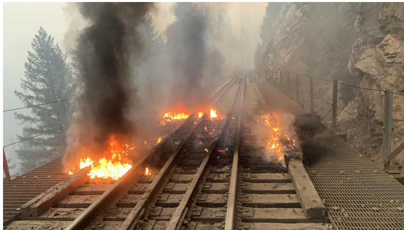
Figure 2.15: Canyon Bridge, Northern California on Fire due to wildfire (InsideTrack News Article, 2021)
