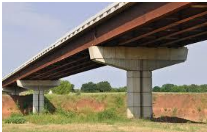
Figure 2.6: Steel Bridges (Kodur et al. , 2013).
