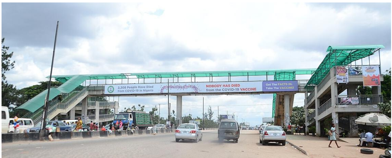
Figure 3. 44 - University of Benin Pedestrian Bridge
