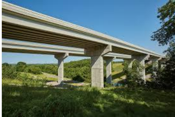
Figure 2.8: Reinforced and Pre-Stressed Concrete Girders (Zhou, & Peng, 2024)
