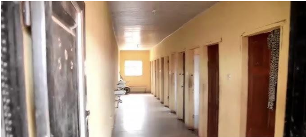
Figure 2.1: The corridor of uselu toilet facility, egor LGA, Edo state.
