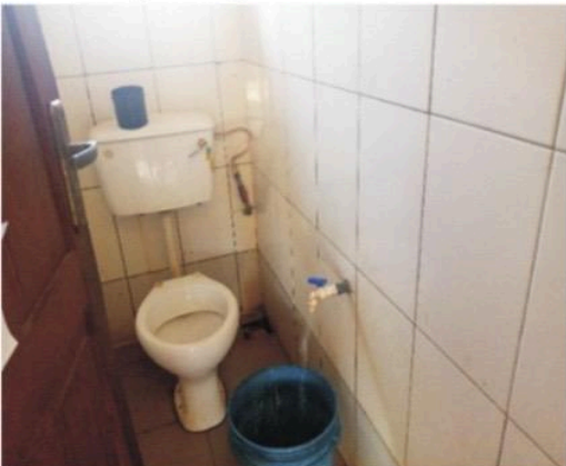
Plate 5: Flush toilet at Ogida toilet facility
