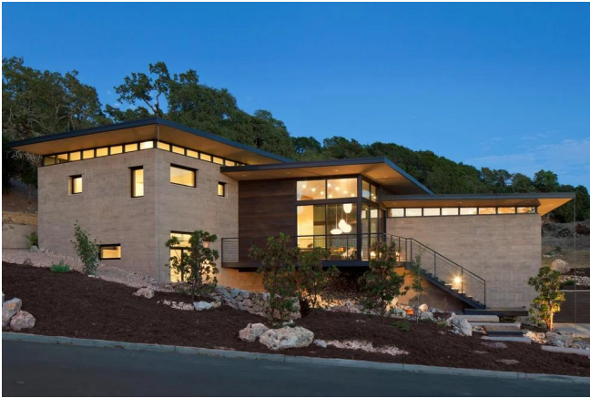
Fig. 2.4. The rammed Napa Valley House in California
