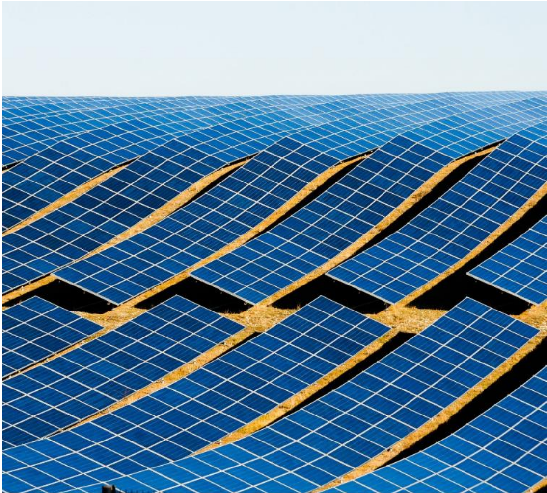
Fig 2.4 Thin Film Solar Panels
