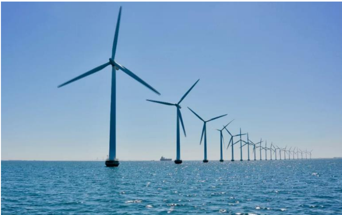
Fig 2.7 Horizontal Axis Wind Turbines
