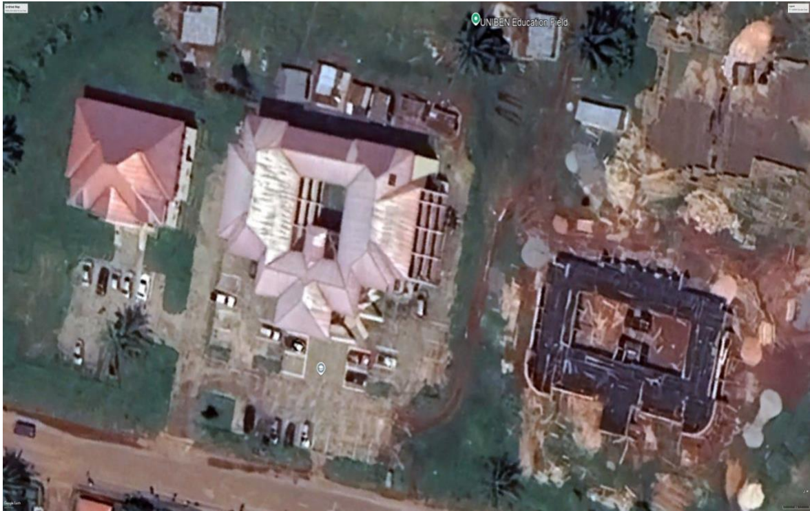
Figure 3.1: Aerial View of Study Area.
