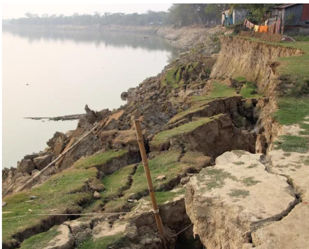
Plate 2.3: Bank erosion in Sunamganj, Bangladesh | Malcolm Dickson/Water Alternatives, CC-BY-NC 4.0
