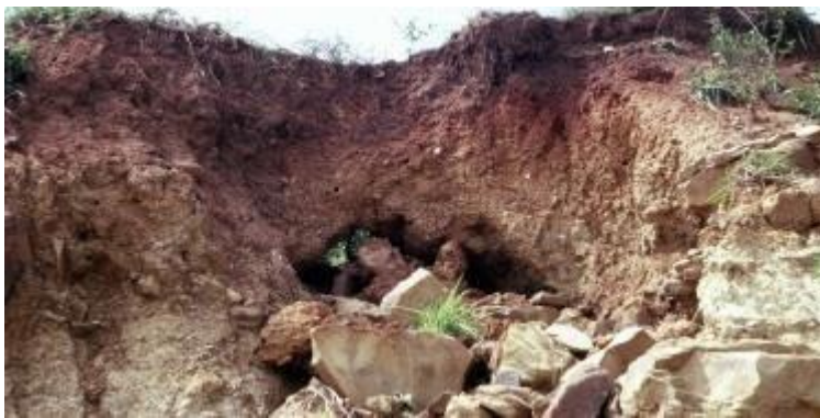
Plate 2.4: Tunnel erosion in Marburg, Queensland (Wikipedia)
