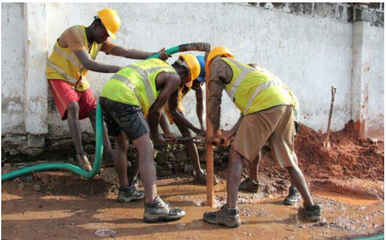
Figure 3. 4: Sludging (Kerstin Danert, 2015)
