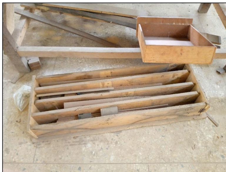
Fig. 3.7 Concrete Beam Mould
