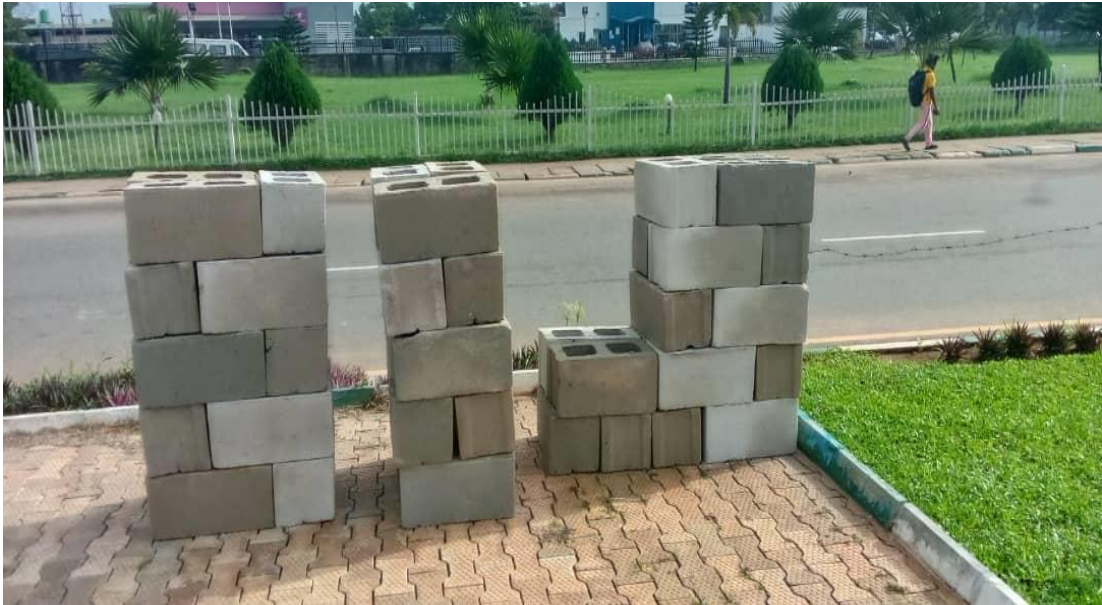
Cement Blocks for the Base of the Graphic Lighting System
