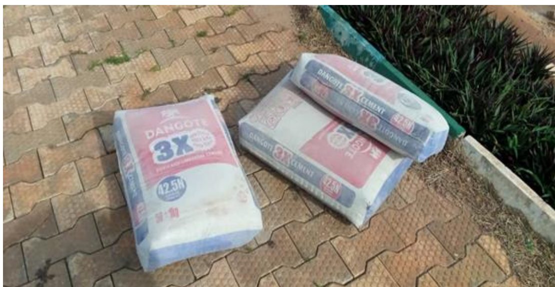
Bags of Cement for the Plastering of the Base of the Graphic Lighting System
