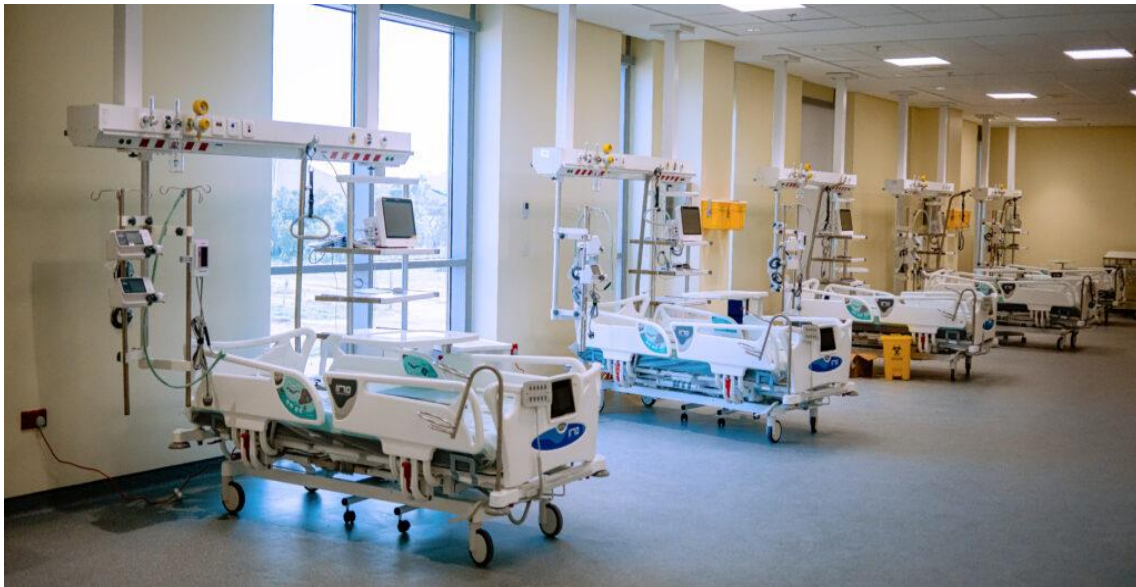
Fig 13. Overview of the facilities in the AMCE, Abuja
