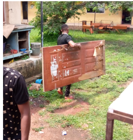
PLATE 9: REMOVAL OF THE OLD DOOR
