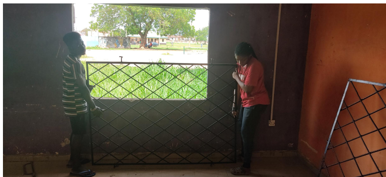
PLATE 5: WORK ON THE WINDOW BURGLARY PROOF
