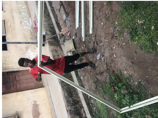
PLATE 3: Coupling Of Aluminium Frames For The Window
