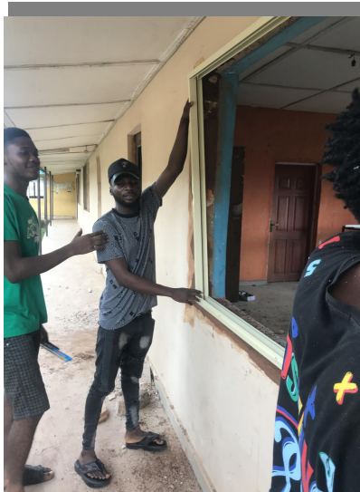
Plate 4: Fitting Of The Frame
