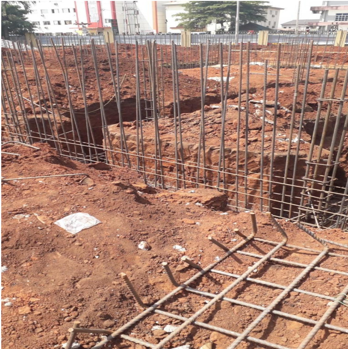
Figure 14: Site of the construction of the storage facility in NCMM, Benin City
