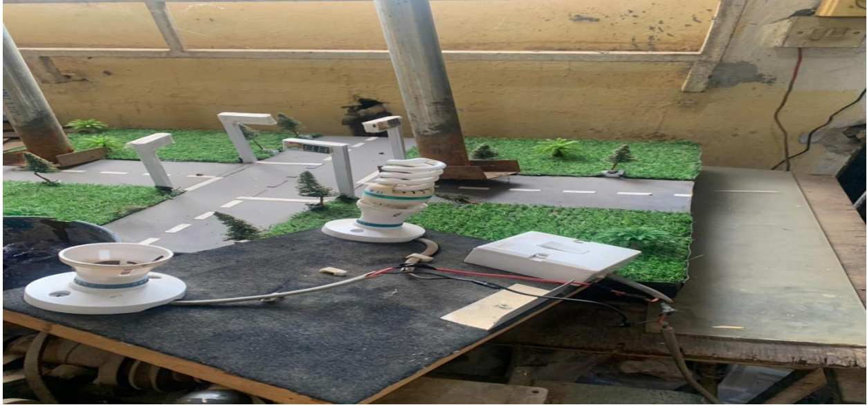
Fig 5.9: AC load in its OFF state connected to the solar system
