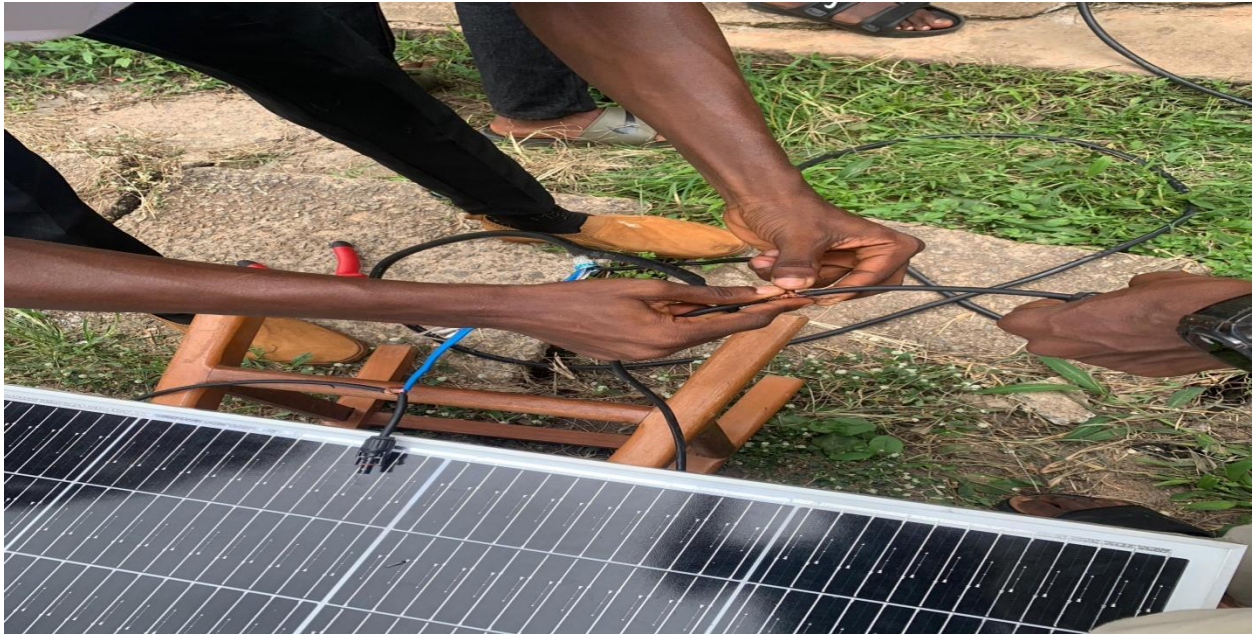
Fig 5.7: A Connection of the solar panel to the charge controller using a solar wire
