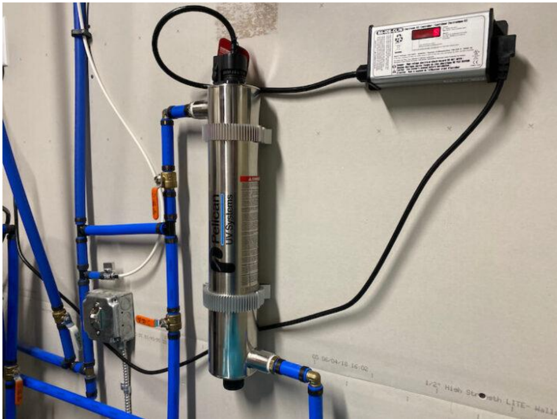
Figure 3.3: UV Treatment set-up
