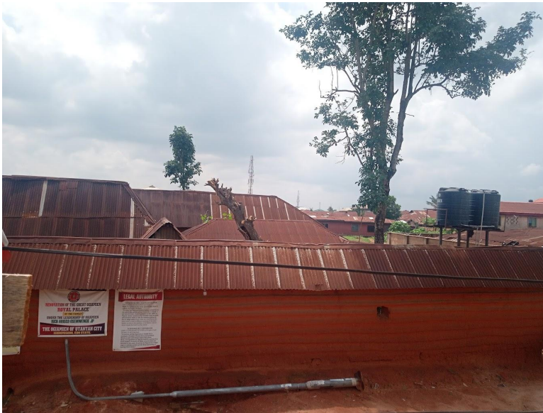
Plate 4.03– Showing the roof used in the Palace
