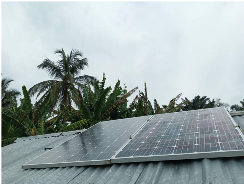
Figure 21: PV panel Installation Process
