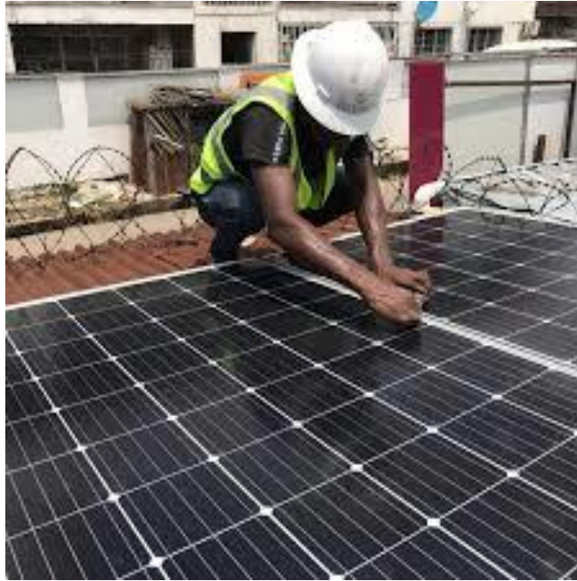
Figure 20: PV panel Installation Process
