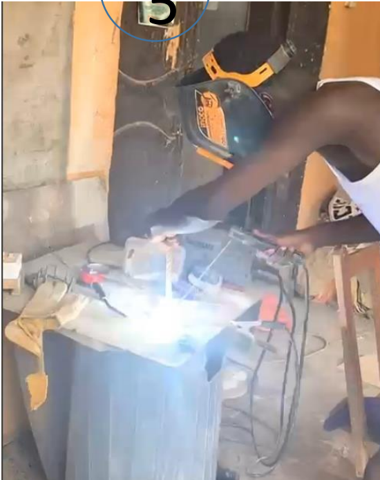
Welding Of hand rails and rudder.
