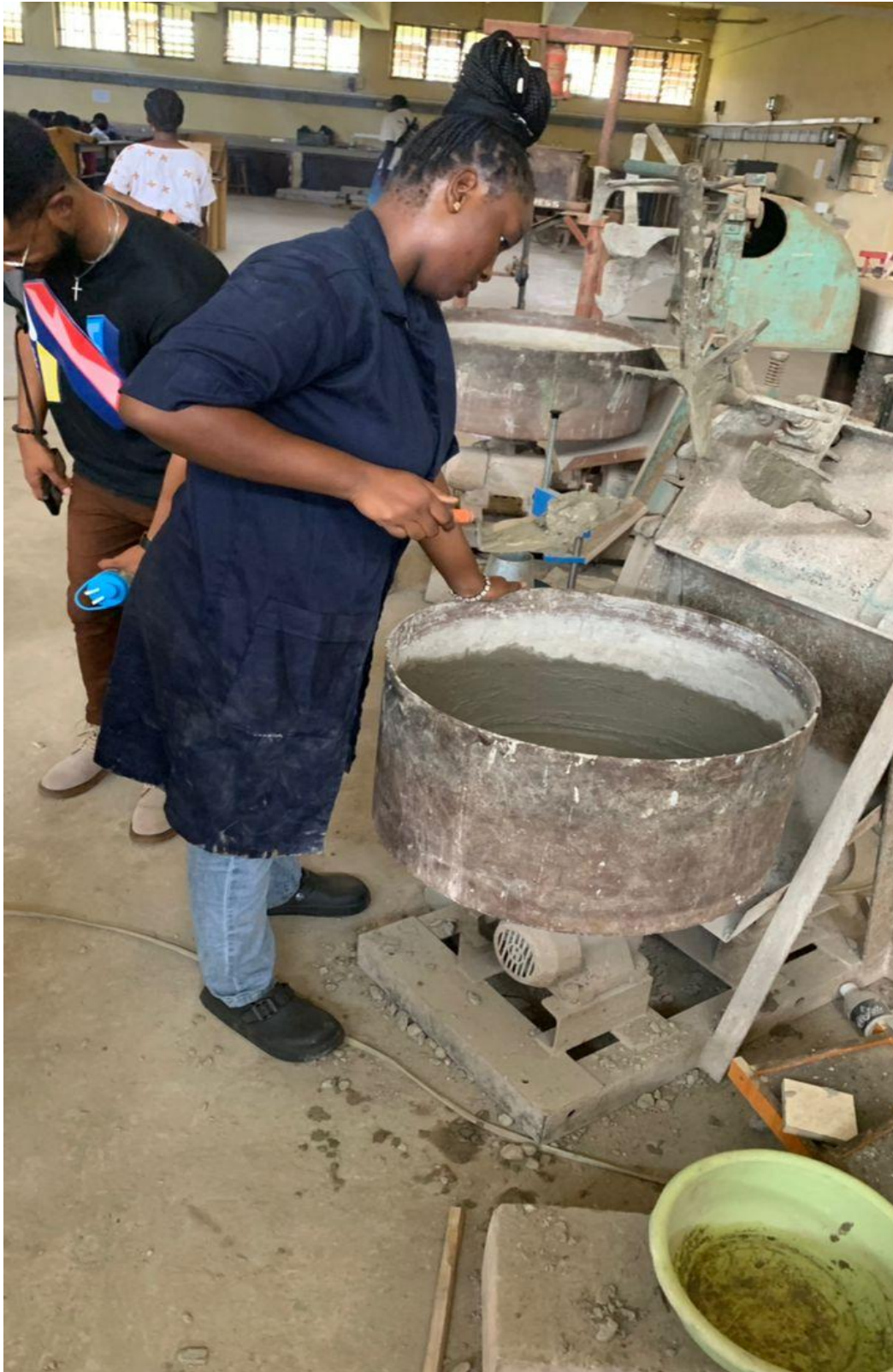
Fig4; Mixing of concrete mix in the concrete mixing machine.
