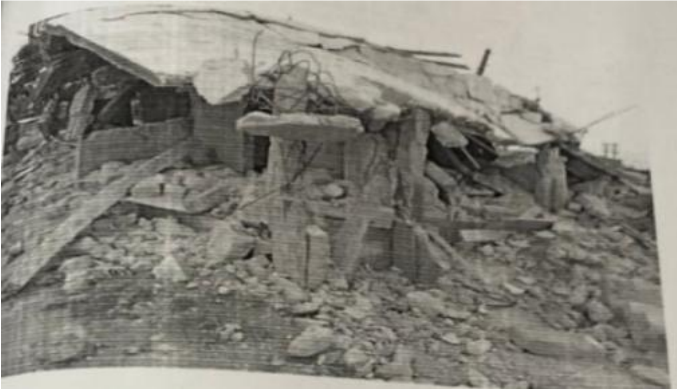
Plate A - 3: Building after collapse
