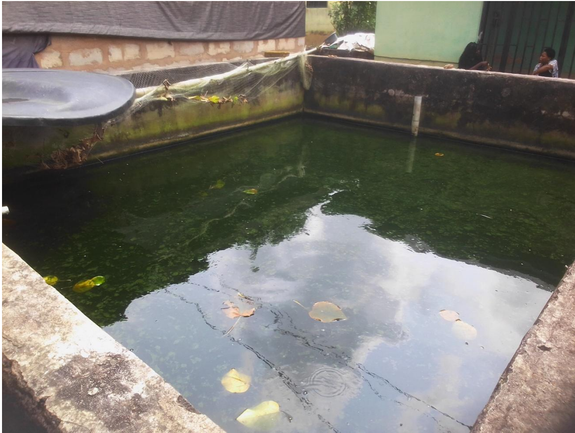
Figure 3.4: pond B which had a 13 – day retention period before water turnover.
