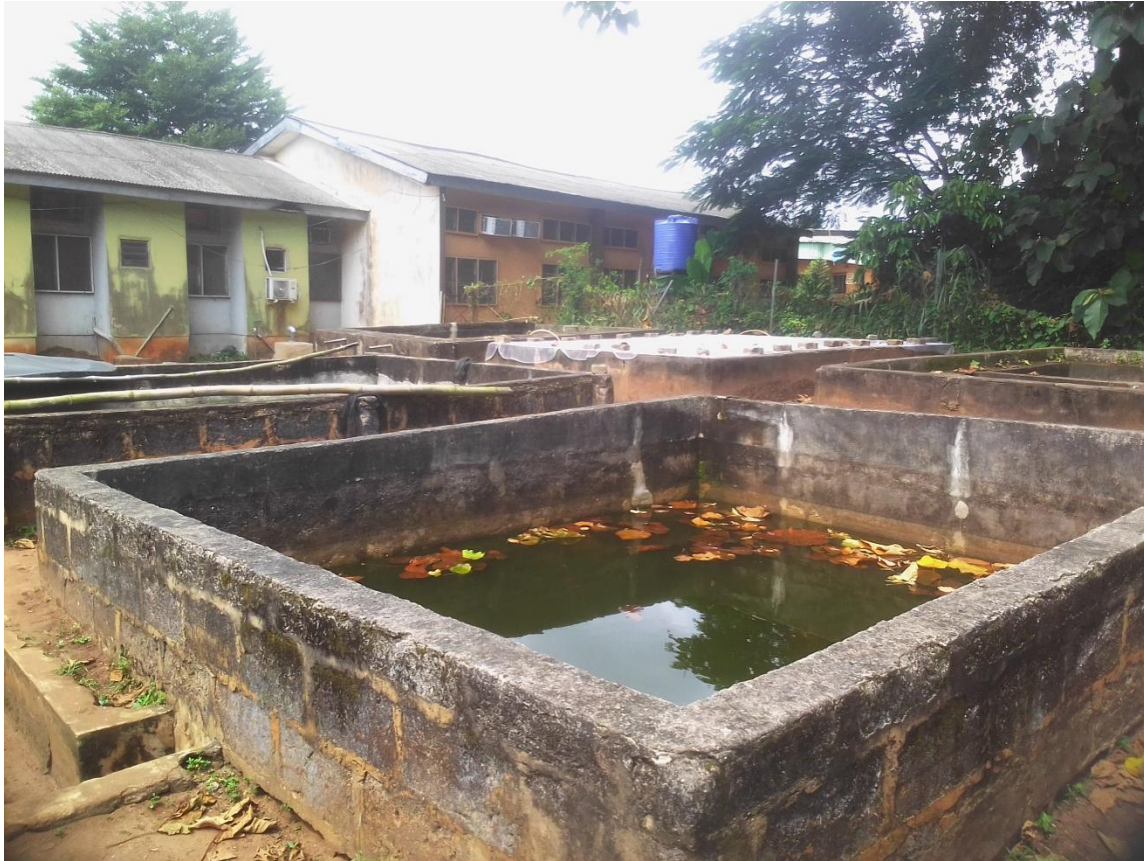
Figure 3.2: fish pond facility at the Faculty of Agriculture
